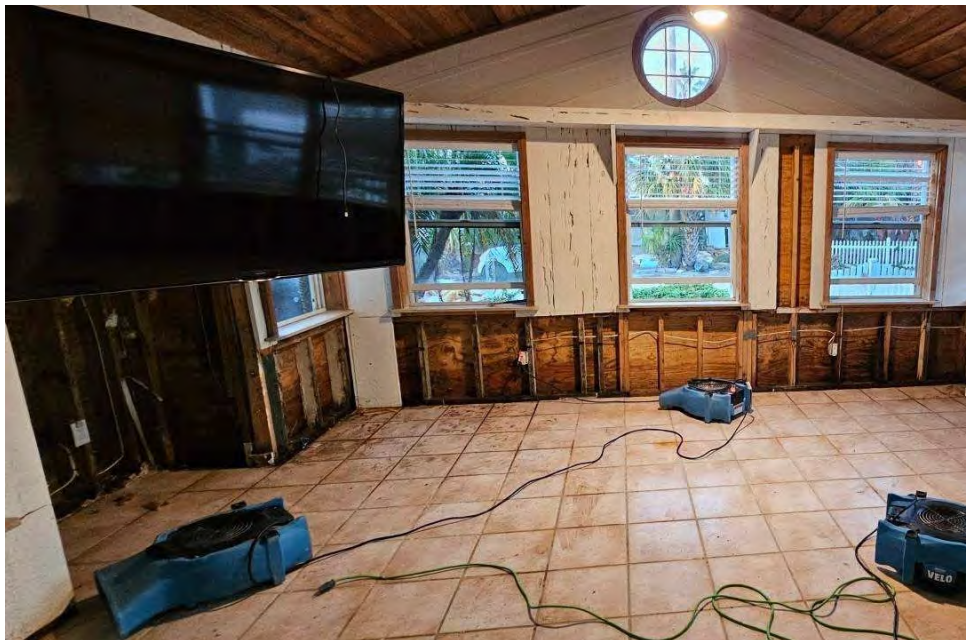
FRONT ROOM AFTER REMEDIATION
