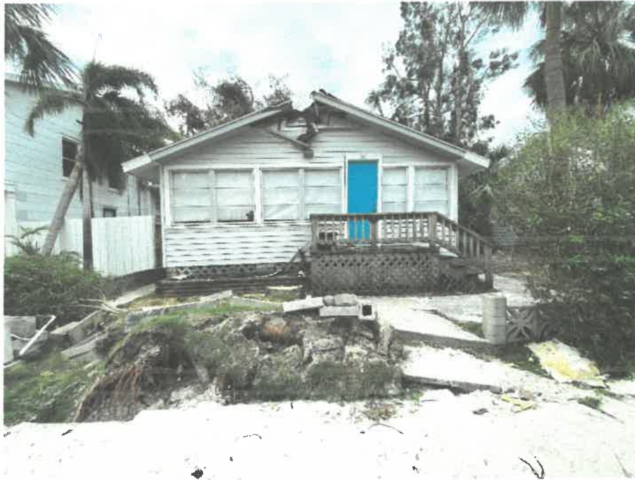
Photo 2: Front View of Building. (North)
