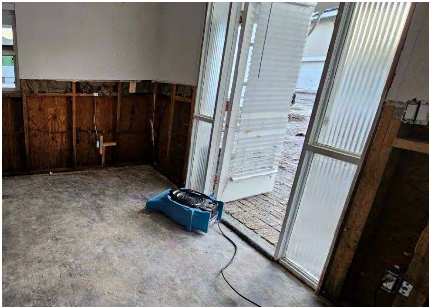
BACK ENTRY AFTER REMEDIATION
