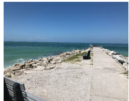
Figure 22: 1 st Avenue Fishing Jetty
