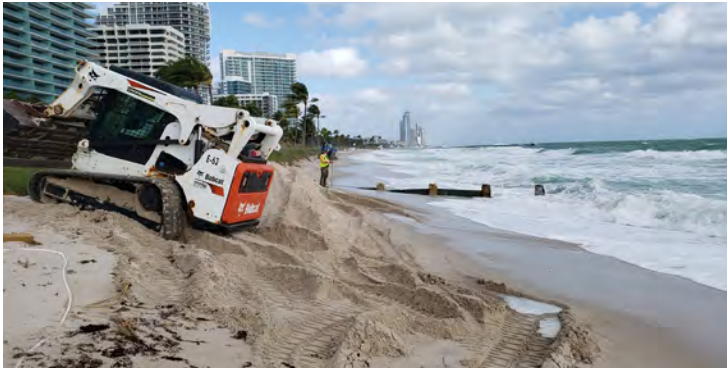
Cummins Cederberg worked with Miami-Dade County to design an emergency dune restoration project following significant erosion associated with nor'easters in 2020. The design was optimized to maximize the fill template while avoiding impacts to nearshore hardbottom.
