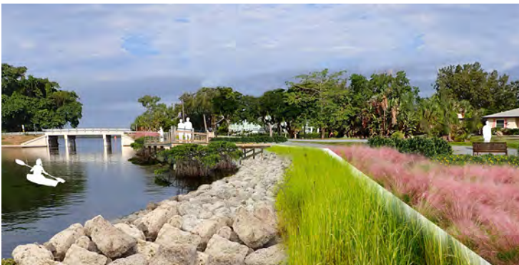
At Portosueno Park in Bradenton, Cummins Cederberg designed a multi-faceted living shoreline that creates environmental habitat, enhances waterfront recreation, and improves resilience with oyster reef balls, mangroves, rock revetment, upland plantings, and an over-water viewing platform
