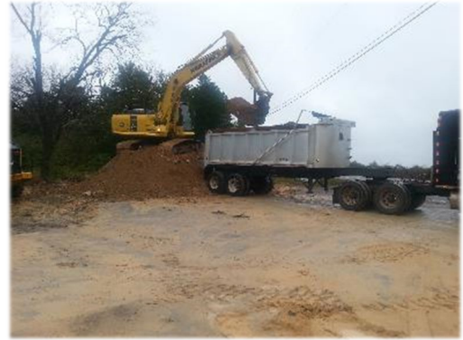
Figure 8: Petroleum-Impacted Soil Removal Along SR 79 During Roadway Improvements
