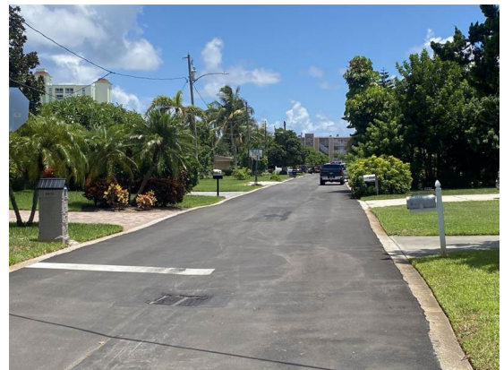
Figure 3: Resurfaced Bay St in St. Pete Beach
