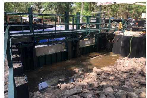
Figure 26: Modified Lake Pretty Structure
