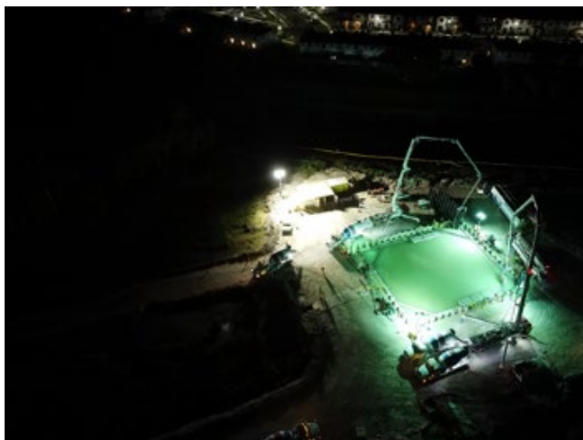
Figure 10: Aerial View of Cutler Pump Station construction
