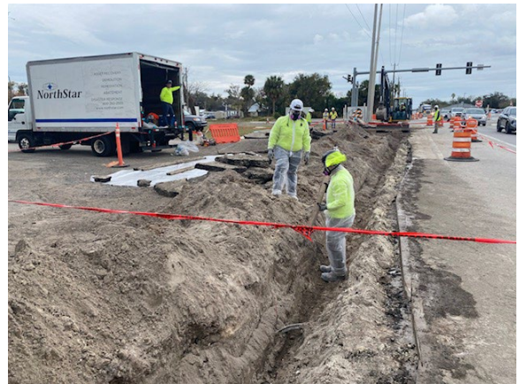
Figure 4: NorthStar Asbestos Abatement Project
