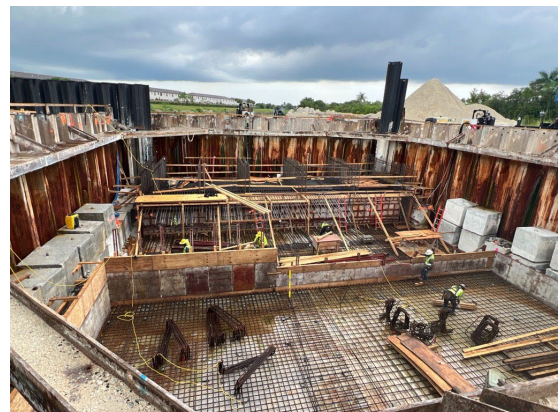
Figure 24: Cutler Wetlands C-1 Flow Way Pump Station Construction
