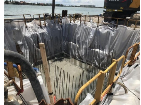
Figure 9: Construction of 3 rd Avenue Stormwater Pump Station in St. Pete Beach
