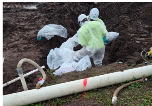
Figure 5: NorthStar Personnel Performing Transite Pipe Abatement On Recent Asbestos Project
