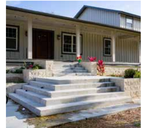
[92] Matching new stairs with the style and features of the historic property is a recommended way to integrate the new foundation and access points. Concrete stairs with landscape planters referencing the new foundation material helps maintain a visual consistency. Photo: p3elevation.com
