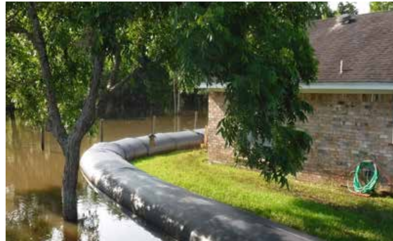
[21] A rural homeowner has deployed a water-filled temporary dam or water bladder to act as a floodwall around their residence. Water bladders require a storage area when not in use and the resources and time to fill them when a flood is imminent. Photo: Aqua Dam, Inc
