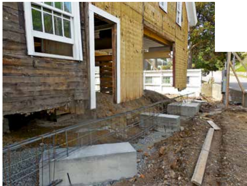
Figure 3: The structure was lifted in sections several feet in the air to provide space and access for foundation work. Photo: GNCB Consulting Engineers
