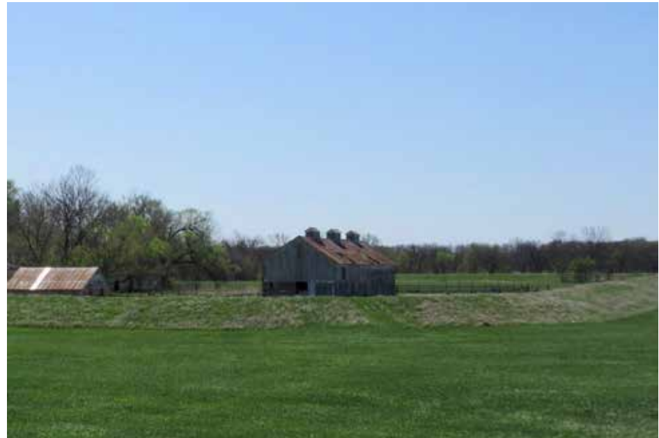
[31] This small-scale levee or berm has provided flood protection to this property in Chase County, KS, since the 1940s. Photo: Steve Samuelson
