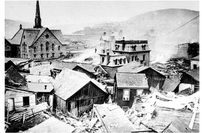
[10] The Great Johnstown Flood of 1889, caused by a catastrophic dam failure, shows the extent of damage that can occur from a large-scale, fast-moving flood event. Whole buildings were destroyed, others were shifted from their foundations, and massive amounts of debris caused considerable loss of life, damage, and destruction. Photo: NPS
