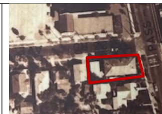
A 1972 aerial of the property, showing the subject structures.
