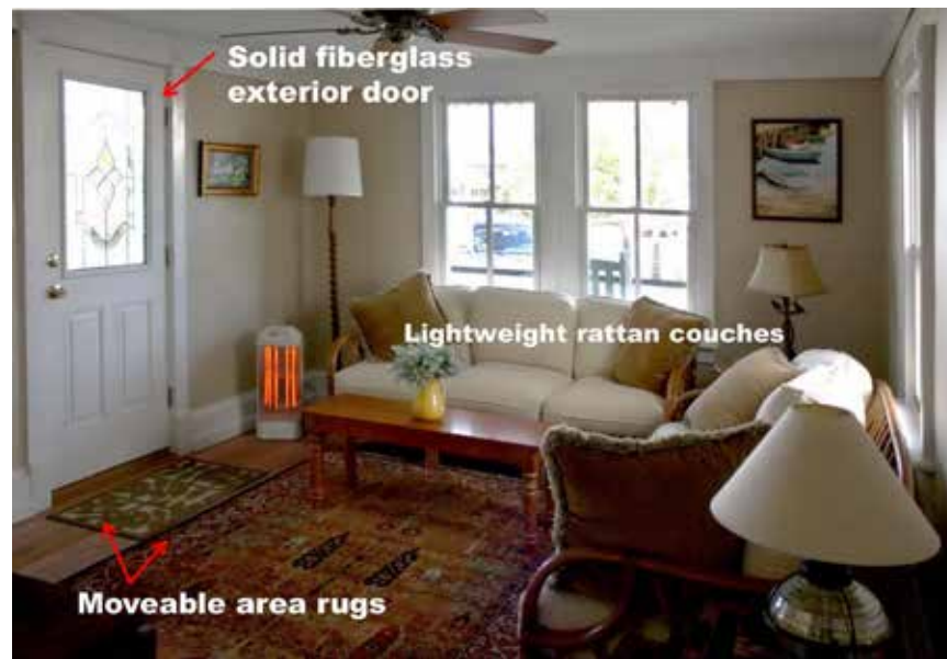
Figure 7: After repairs and wet floodproofing measures have been implemented, the new floor and wall surfaces are flood-damage resistant. The front door and windows were also replaced with more compatible designs using flood-damage resistant materials Photo: Mary Delaney Krugman, JD, MSHP
