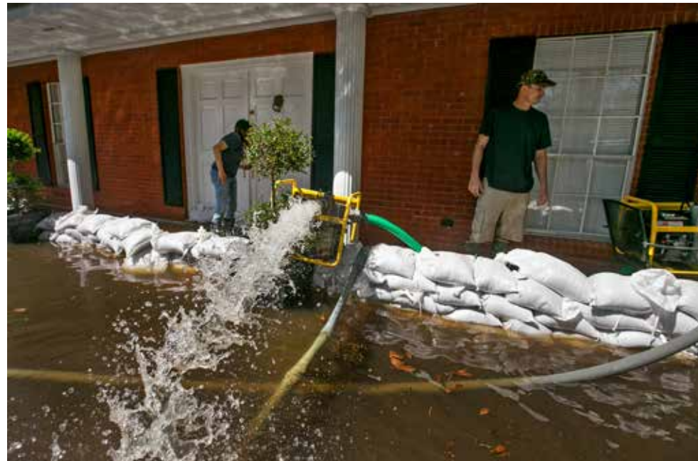
[26] Water can still seep through sandbag barriers. A property owner should have a pumping system with back-up generators to remove water from behind the barrier. Photo: Ted Jackson, NOLA.com | The Times-Picayune. The Advocate, 7/29/2019. The Times-Picayune/The Advocate
