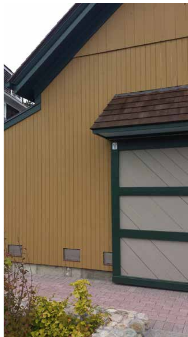
Figure 7: As part of wet floodproofing the building, engineered vents near the bottom of exterior walls are designed to allow water to flow in and out of the building during a flood. This allows water pressure to equalize on both sides of the wall and reduce stress to the structural system. Photo: Jennifer Wellock/NPS
