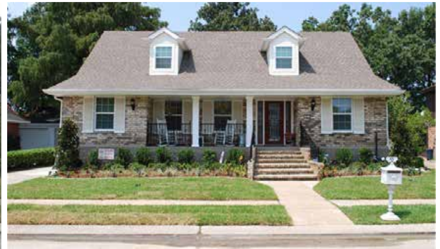
(b) Photo: Rubion Construction Co., LLC
