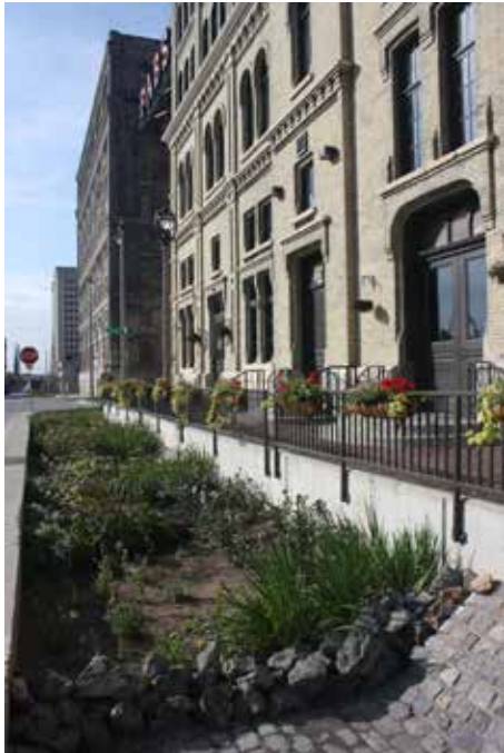
[39] Street and sidewalk improvements that include bio-swales or other water retention systems can be effective devices to collect or direct water and alleviate flooding as shown here in Milwaukee, WI. Photo: Liz Petrella/NPS
