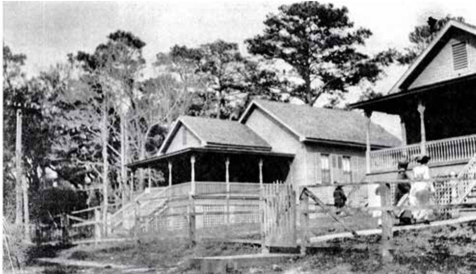
Figure 1: A Queen Anne house (center) on its original site facing Biloxi Bay before 1918. Photo: Robert and Willene Dunnaway Friar/Courtesy of Ocean Springs Archives
