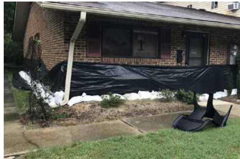
[23] A combination of different temporary measures can be an effective short-term solution to flooding. In this case, a building wrap of waterproof fabric is anchored by sandbags. Photo: Chapelboro.com
