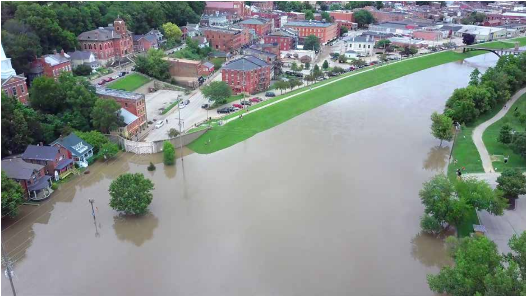
[19] Community-scale interventions, such as this combination of a flood wall, levee, and floodgates in Galena, IL, can protect multiple historic resources and maintain the character and integrity of entire historic districts and neighborhoods. Photo: GalenaGuide.com
