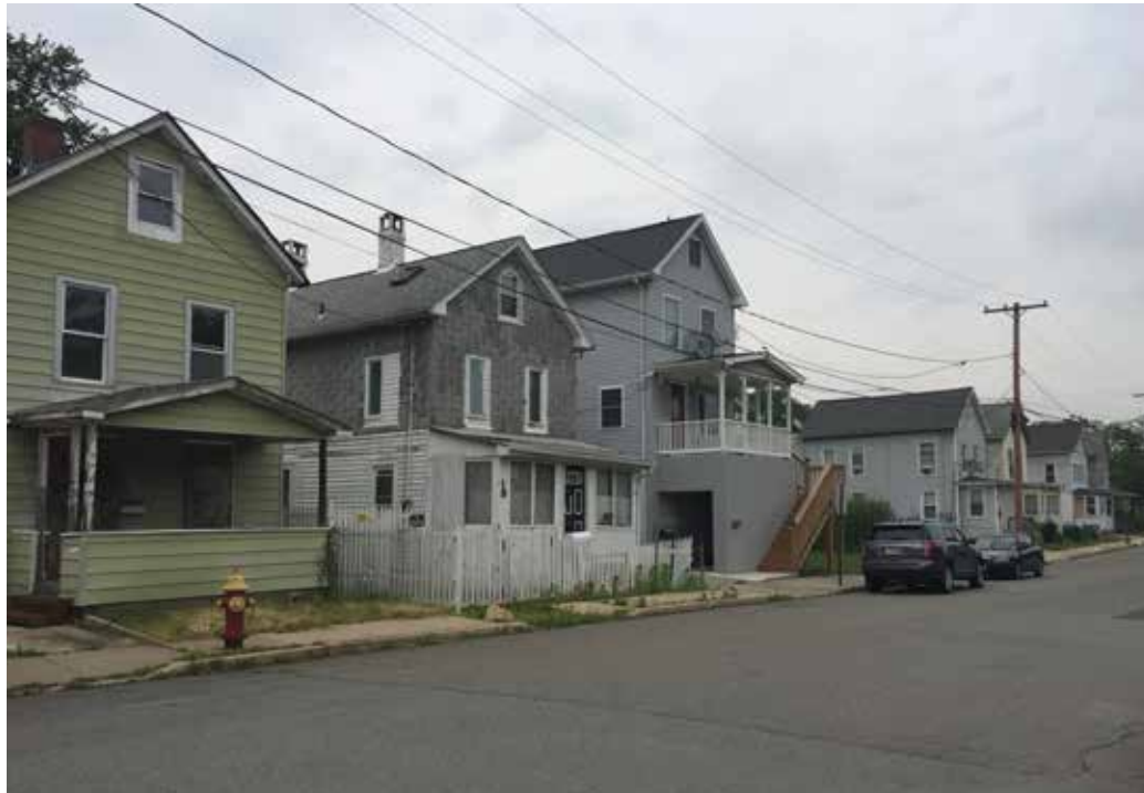
[99] Consideration should be given to the overall impact on the historic character and appearance of a district. A significantly different or random change in foundation height is inconsistent with the historic character of this district. Photo: Jennifer Parker/NPS
