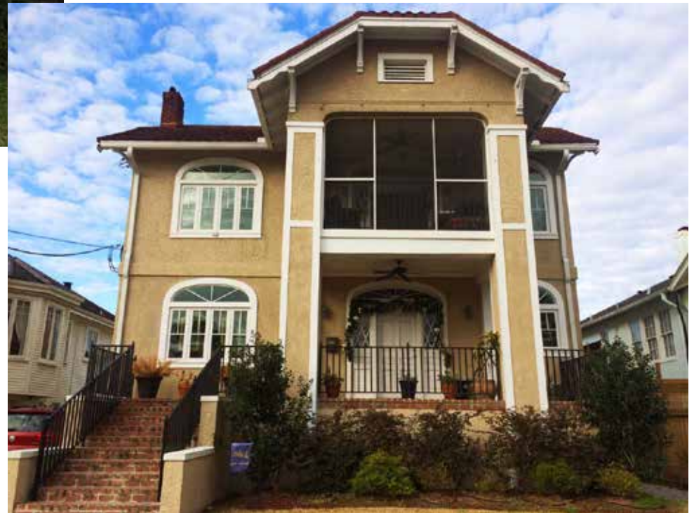
(b) Photo: Rubion Construction Co., LLC
