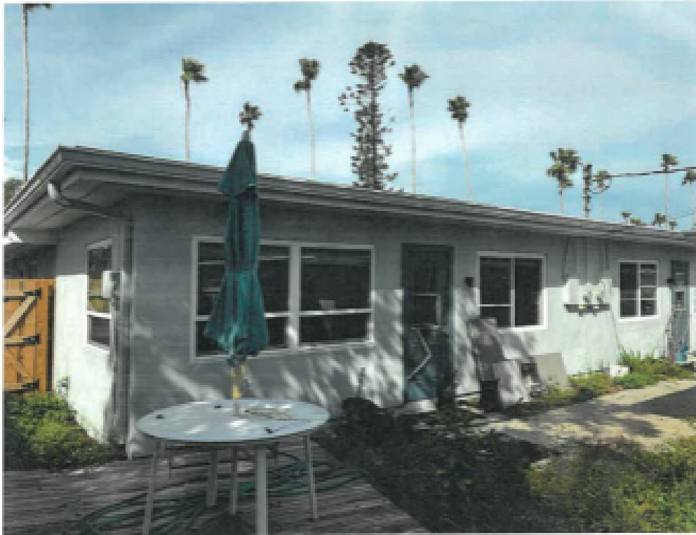
Rear View of East Unit
