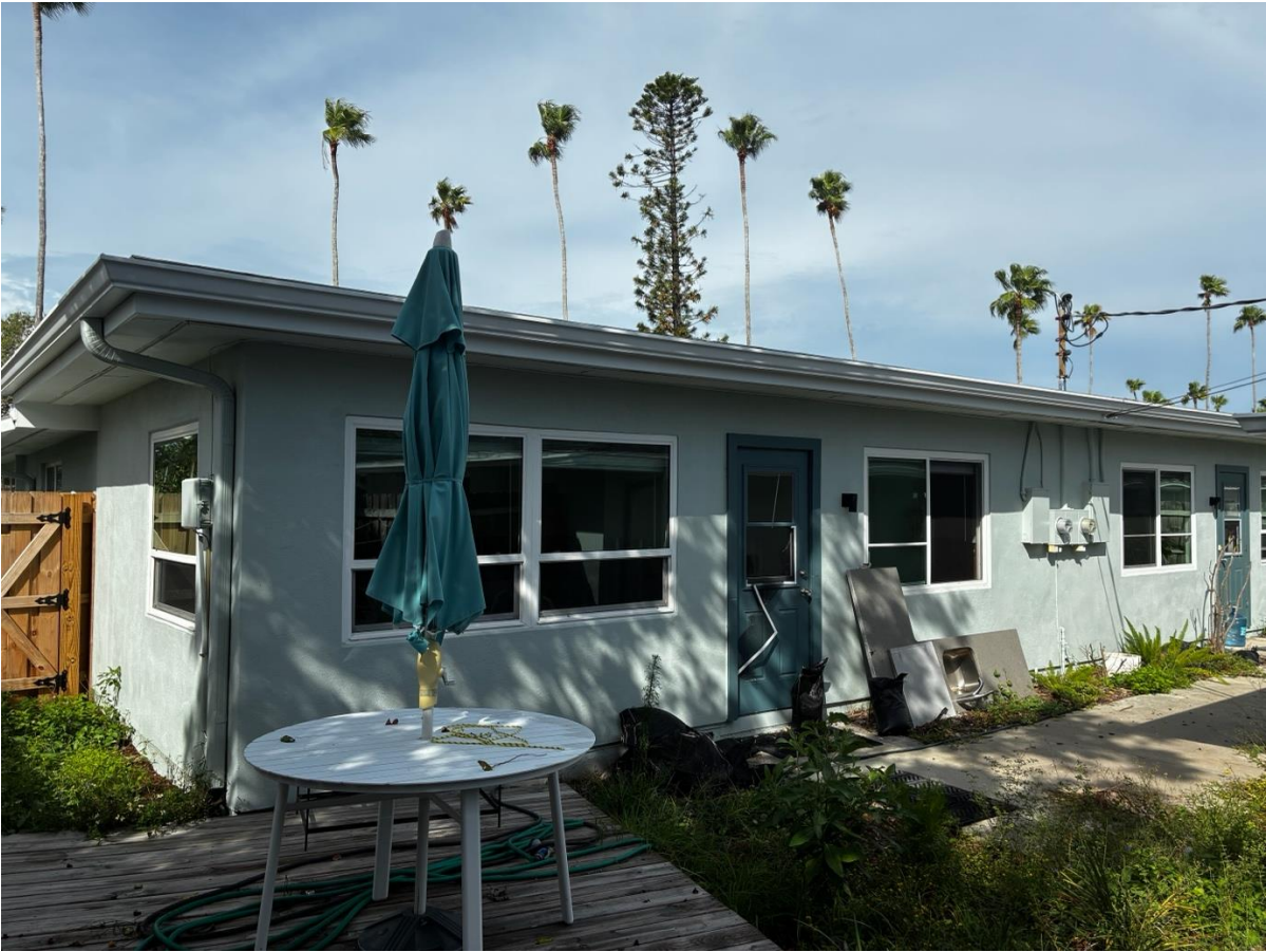
Rear View of East Unit
