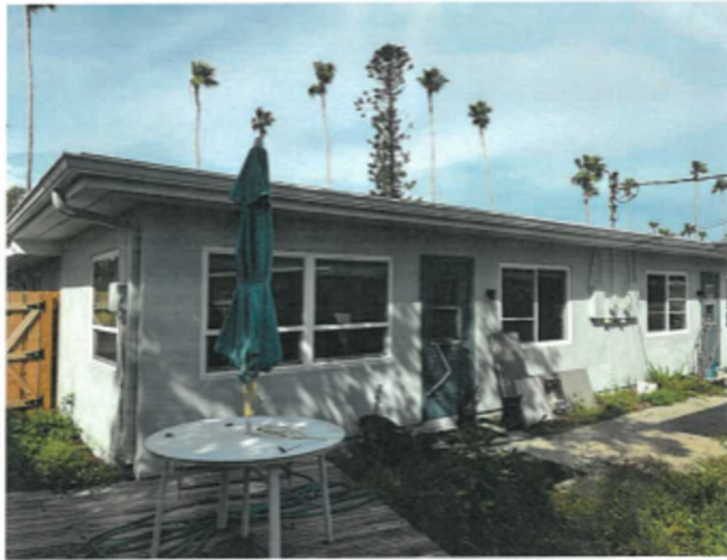
Rear View of East Unit
