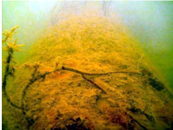
Exposed 18-inch Force Main
