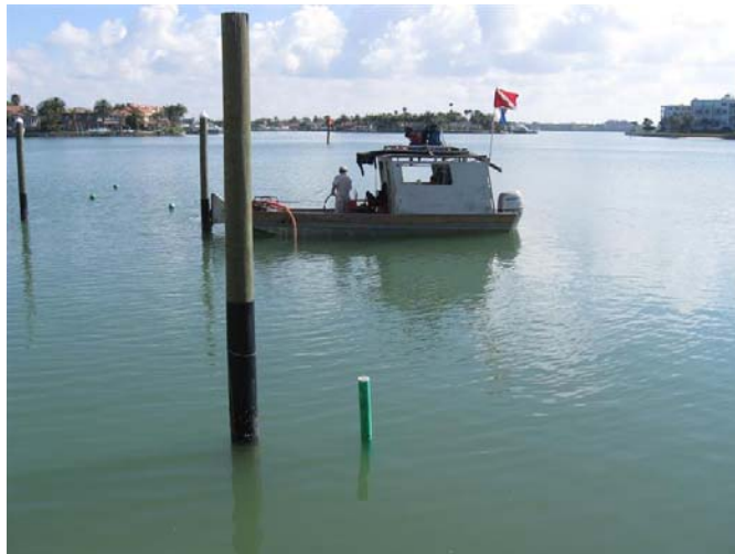
Pilings by Force Main Markers
