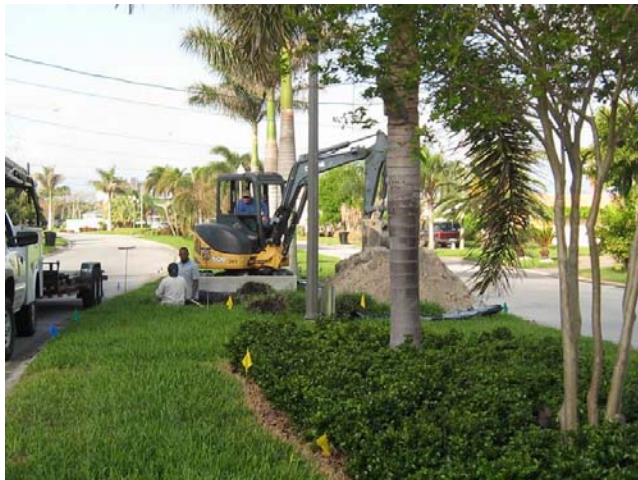
Force Main Excavation along 79 th Street
