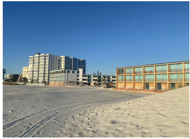
Figure 20 St Pete Beach Dune Damage
