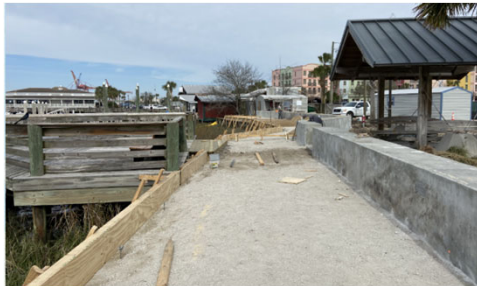
Boardwalk and Seawall Repair (Amelia River Waterfront CRA)
