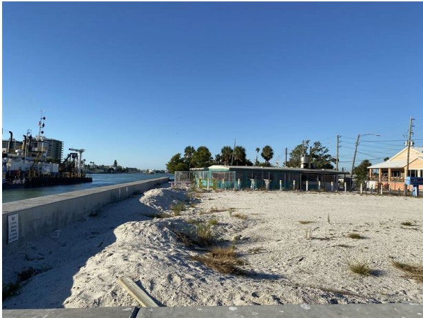
Figure 26 Historic Woody's Restaurant, Severely Damaged and Closed. Sunset Beach.
