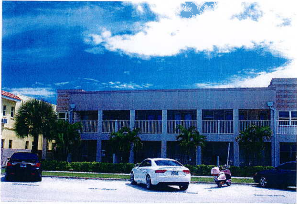
701Gulf Way- Beach Club at Pass-A-Grille West Elevation Facing Gulf Way
