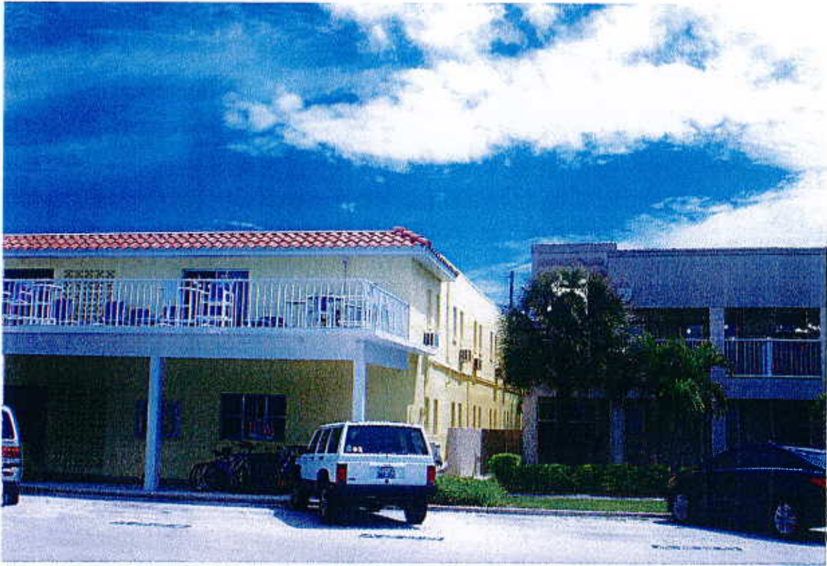
View Looking East Showing Concrete Wall Separating 701 & 709 (PAG Beach Motel) Gulf Way
