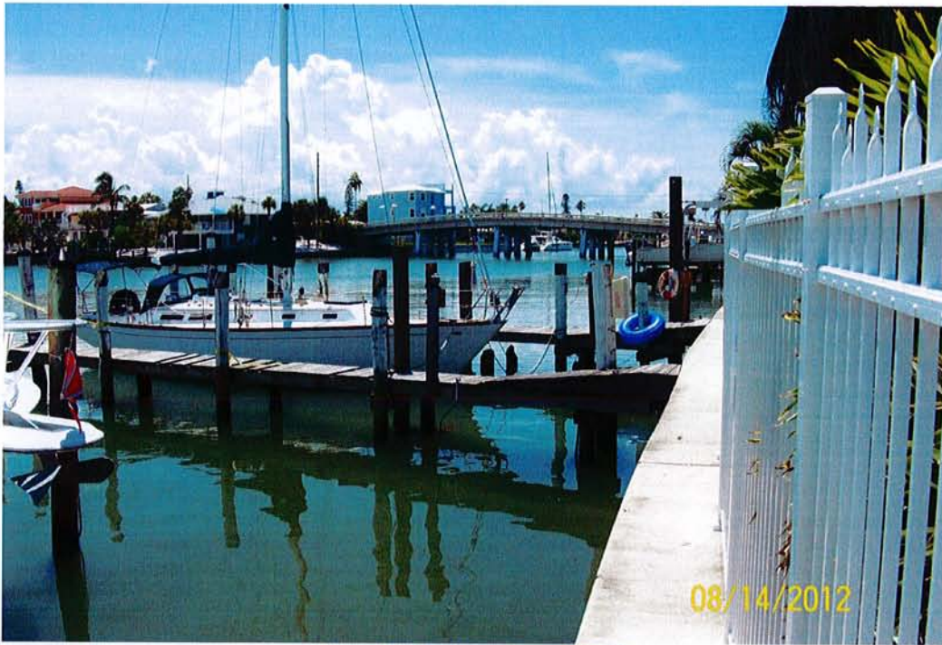
Figure 3. View Along Seawall South
