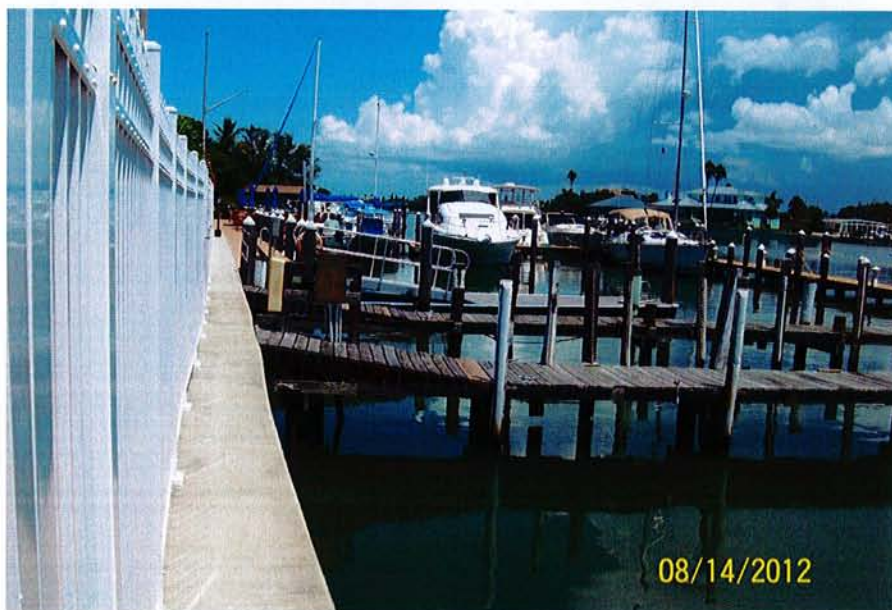
Figure 2. View Along Seawall North
