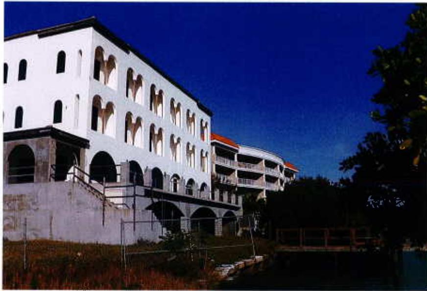
Figure 3. Rear yard waterside
