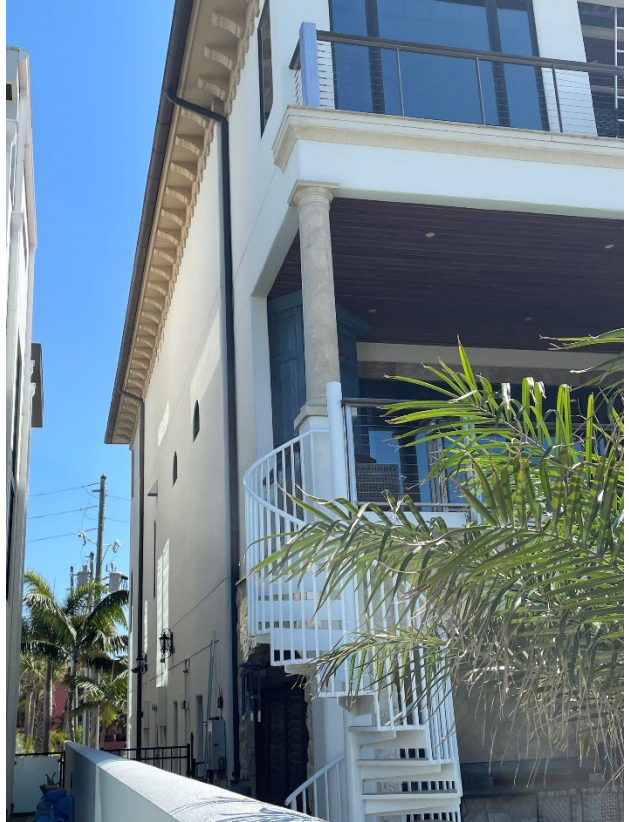
Rear of dwelling and side yard (north) elevation for the proposed generator location
