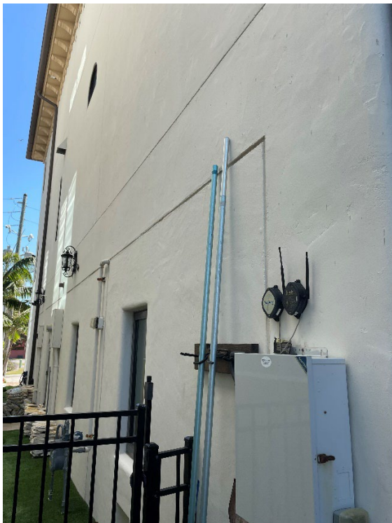
Area of proposed elevated generator
