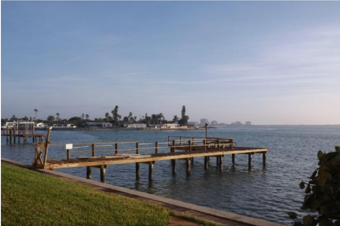
Figure 2. Storm Damaged Dock at 1505 Pass-A-Grille Way
