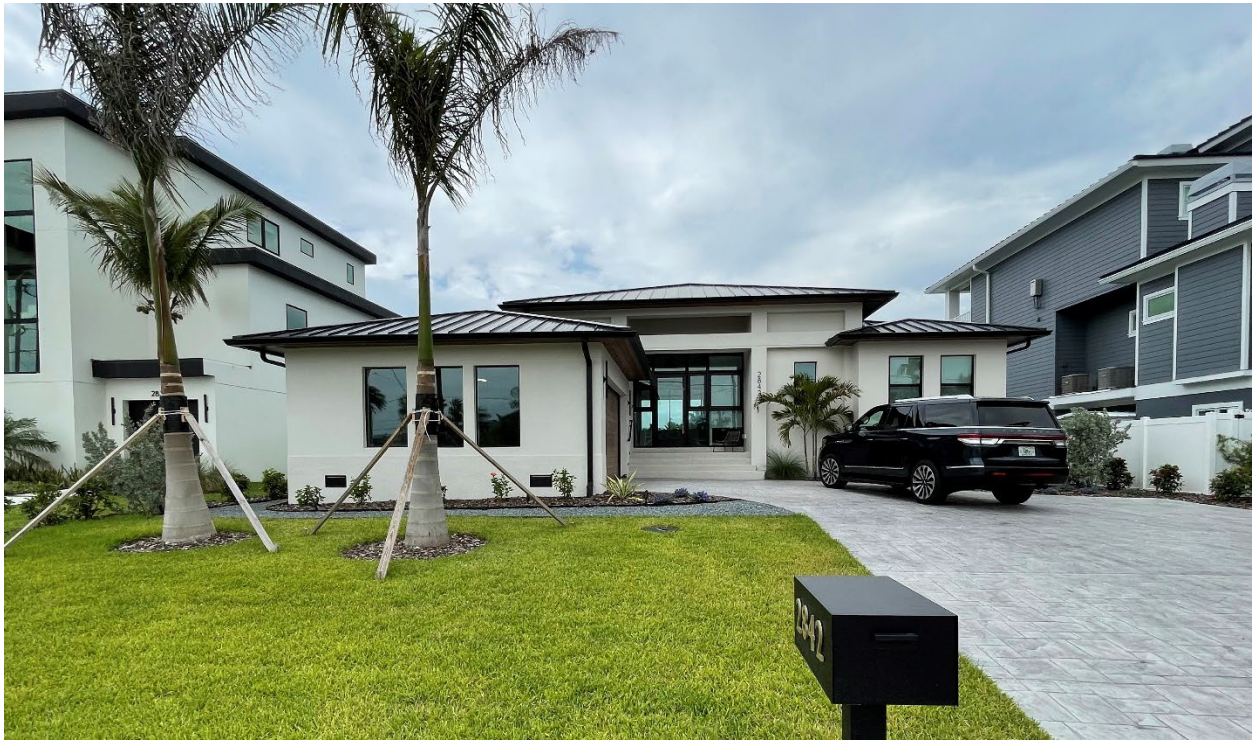
Front of dwelling facing W Vina Del Mar Blvd.
