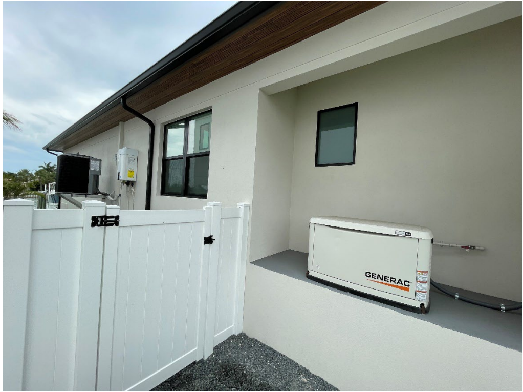
Portion of side yard (south) elevation with installed elevated equipment and generator alcove
