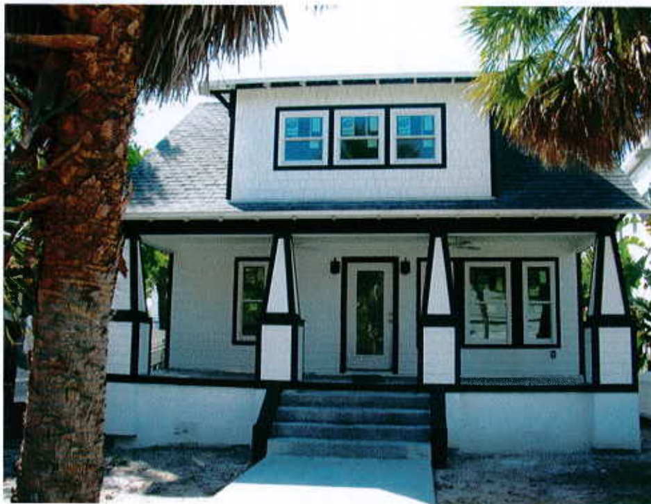
Figure 2: 104 7th Avenue after rehabilitation, August 2012
