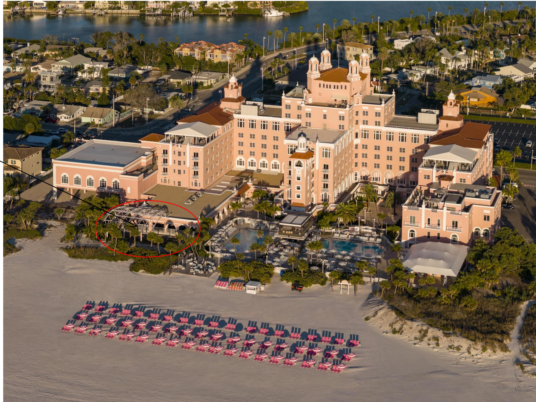
AERIAL VIEW OF THE DON CESAR FROM THE WEST
