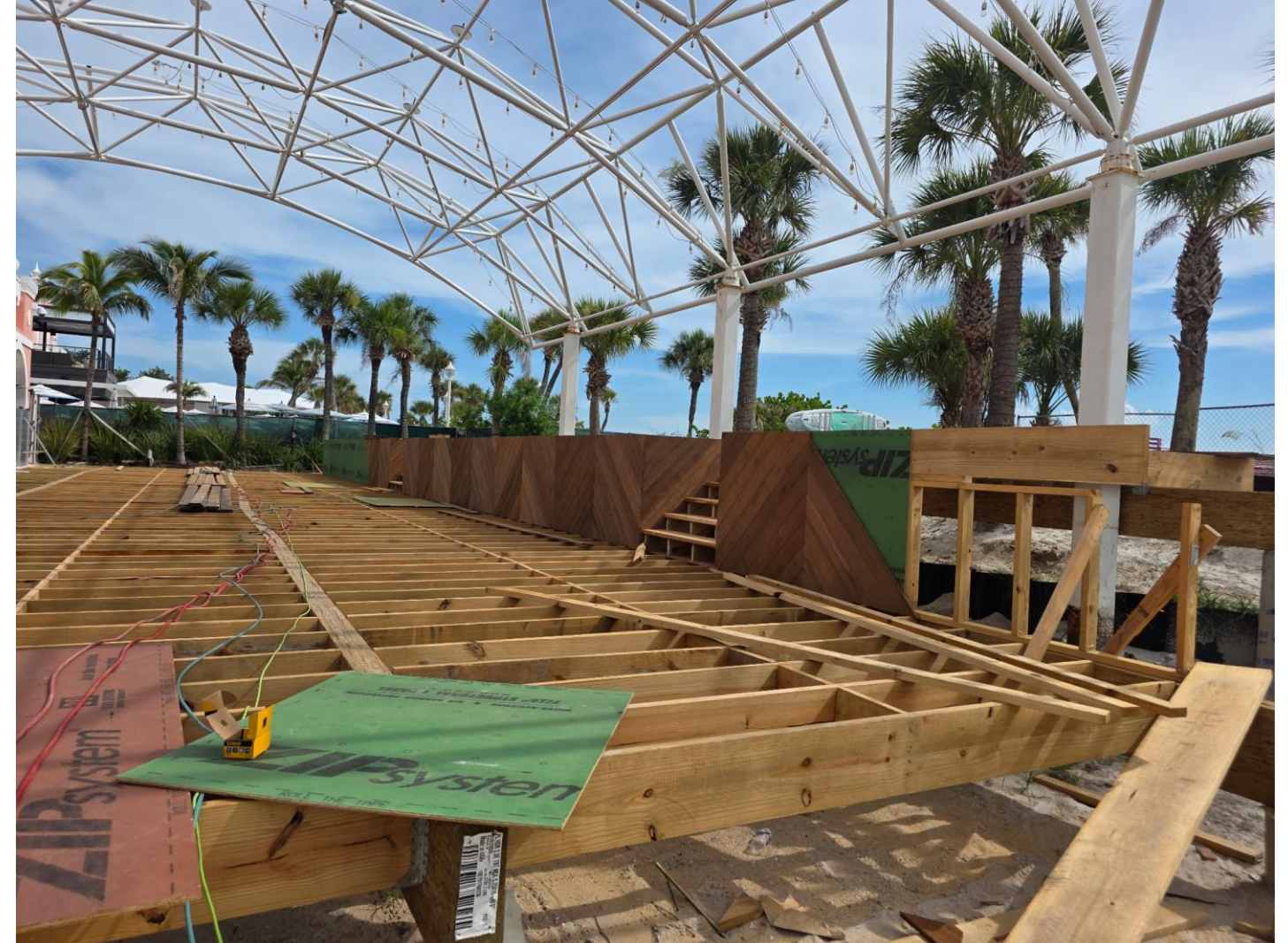
DECK CONSTRUCTION COVERING POND (AREA SHOWN IS NOT PART OF VARIANCE)
