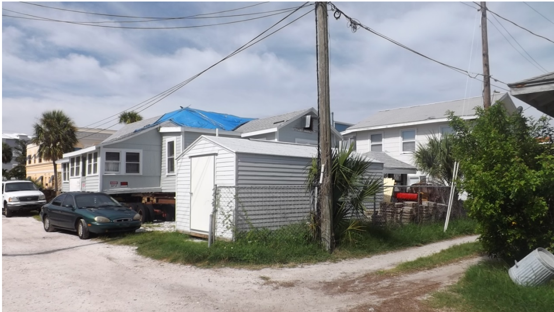
Figure 5. From rear toward 8 th Avenue
