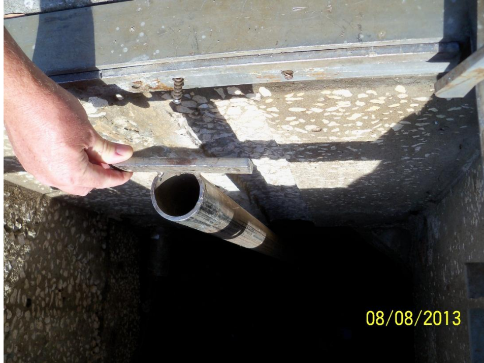
Figure 10 – LS#10 Detached Rail System
