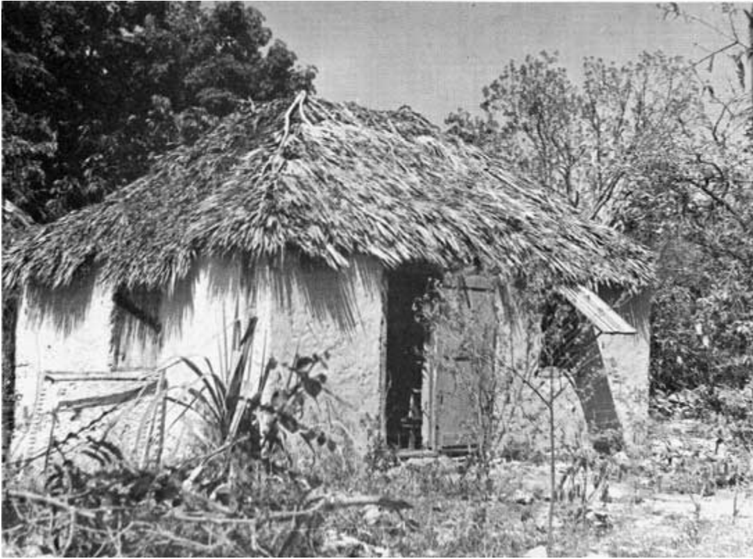
A typical 19 th -century Bahamian cottage with hipped roof thatched with palm fronds, stuccoed exterior, plank door, and top-hinged shutters. Source: Islands in the Sun: A History of the Bahamian People , Vol. 2, page 174).
