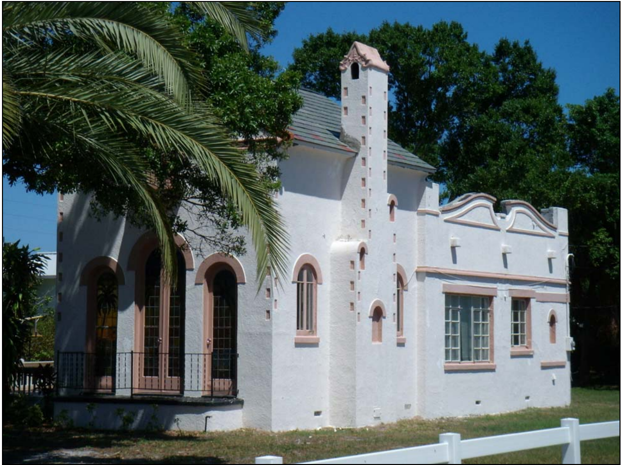
Figure 8 Jules Frere House, 2404 Sunrise Boulevard, Fort Pierce
