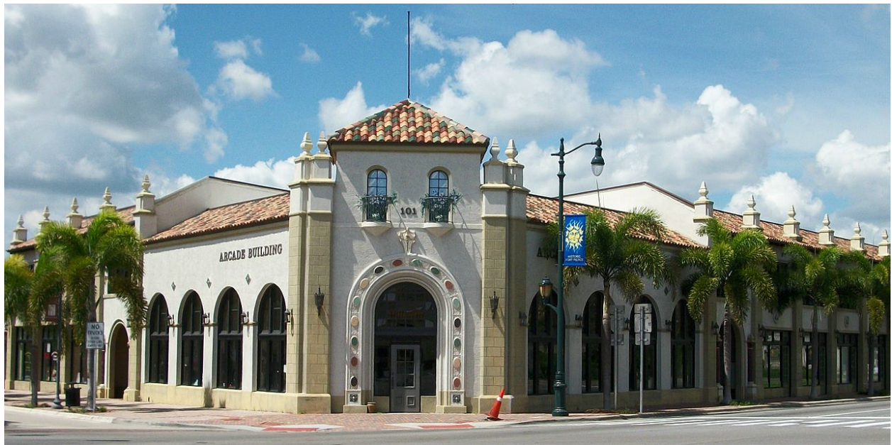
Figure 11 Arcade Building, 101 US Highway 1, Fort Pierce
